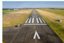
Airfield surface works
